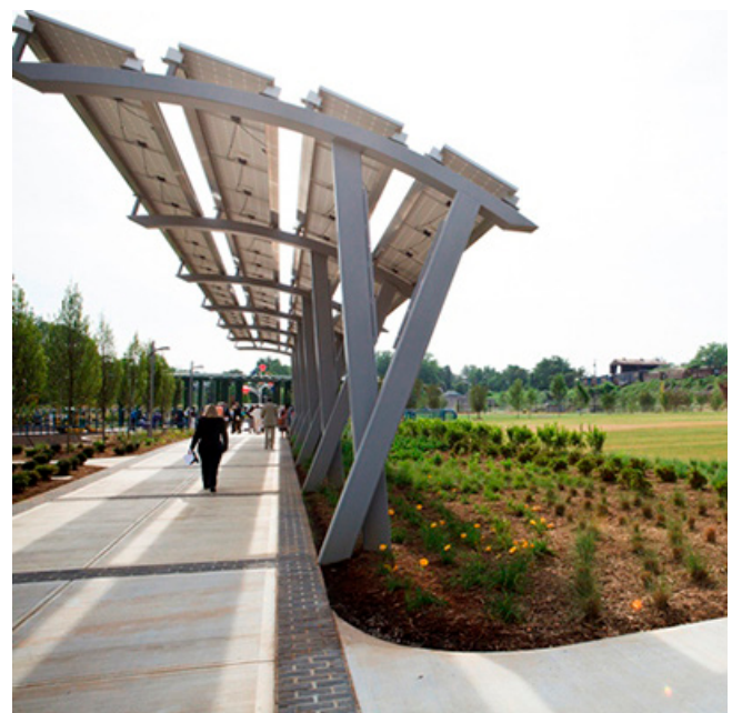
Shade structure with integrated solar, Atlanta Beltline
