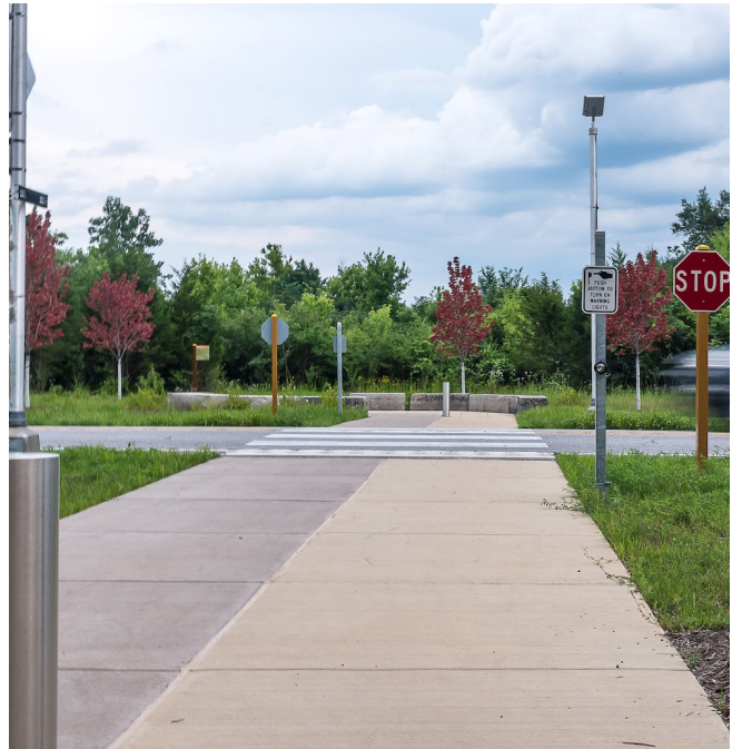
Street crossing condition
