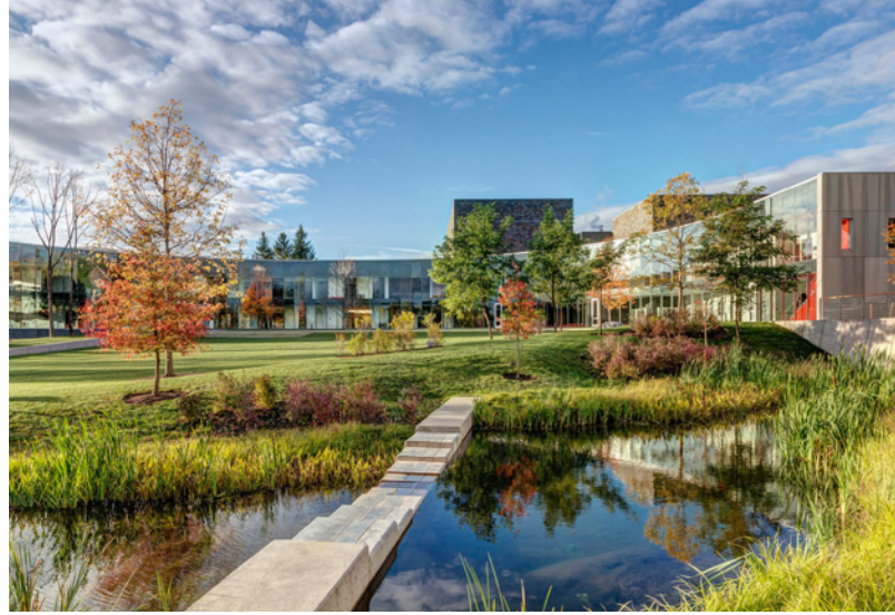
A retention pond with planted, naturalized edges serves as both a landscape amenity and stormwater management.
