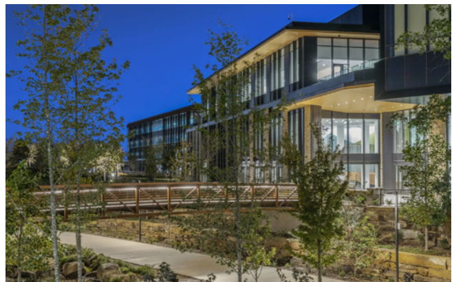
Buildings in RTP should feel intimately and purposefully connected to the landscape.
