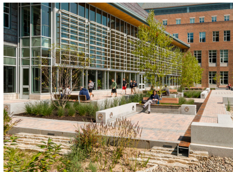
Bioretention and stormwater conveyance integrated into pathways seating areas.
