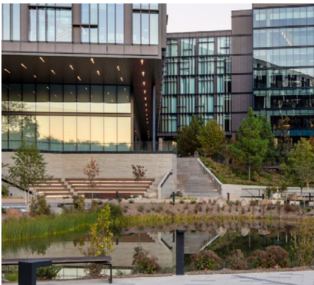
Retention basin as a feature in the landscape with layered plantings and pathways.
