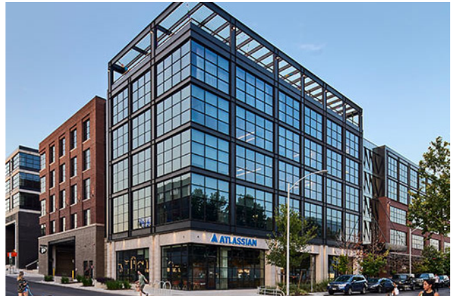
Simple building forms with flexible floorplates and convertible ground floors are more adaptable and future-proof.
