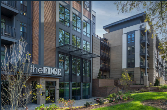
A multi-family residential building in Winston-Salem featuring a natural, earthy material palette and subtle color shifts.
