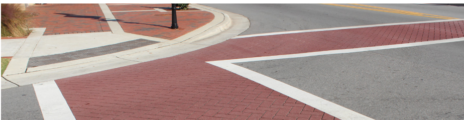
Crosswalks: Typical stamped and surface coat treated asphalt. Surface color applied with Endurablend or equal product.
