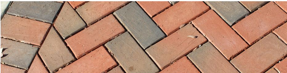
Typical permeable brick paver in herringbone pattern and single soldier edge course in furnishing zone of streetscape.
