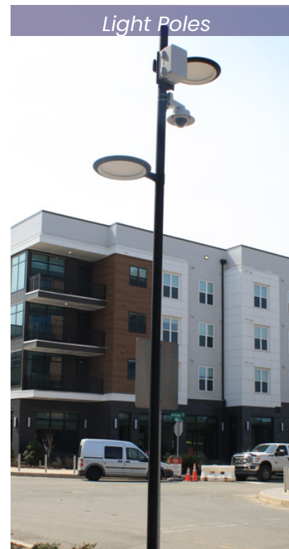
Example of a consolidating lighting, camera, and Wi-Fi infrastructure to reduce poles, RTP HUB (Source: Kimley-Horn)
