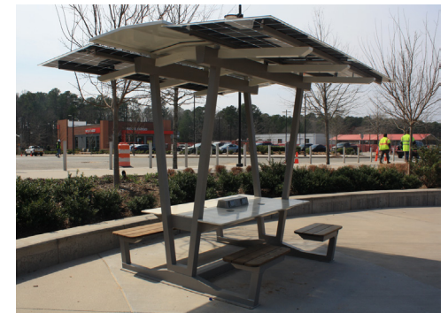
Example of a picnic table with solar panels powering 120 volt power sources. (Source: Kimley-Horn)
