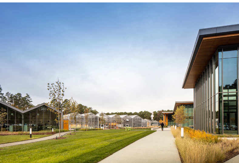
Alexandria Center for AgTech in the RTP shows a move towards ECC-style development with a pedestrian focused core, trail connections, and restaurants.
