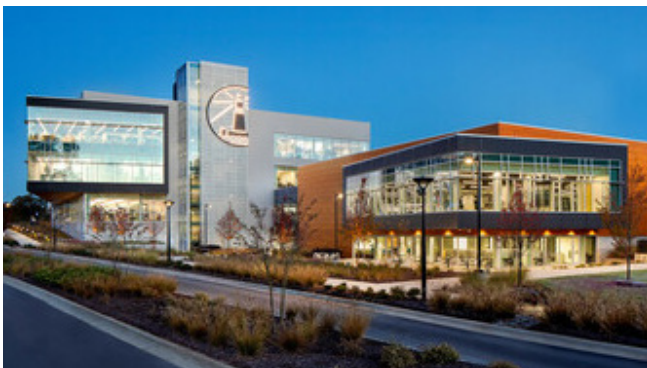
Recent RTP development incorporating enhanced connectivity and on-site amenities for employees.
