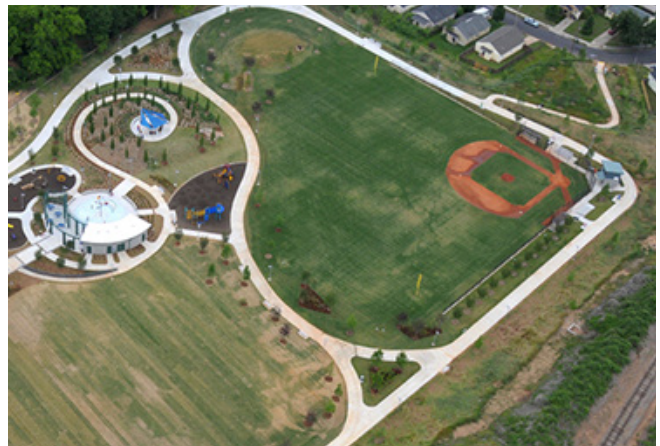
This public park and recreation field adjacent to the Atlanta Beltline is a regional amenity.
