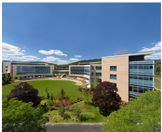
Regeneron BioMed Realty Campus in Greenburgh, NY maximizes natural light and connections to open space through its compact, walkable footprint.
